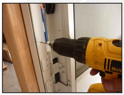
Pre drill mounting screw holes using + - .095" bit.
