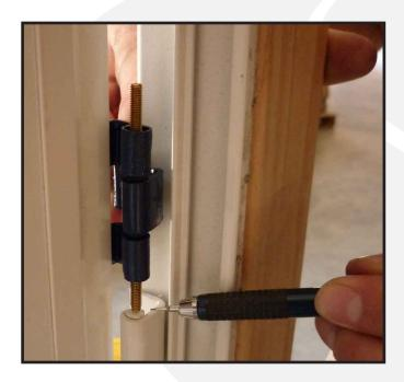
Using a HAC installation /mounting template, locate the center of the existing hinge. This aligns the pivot centers for a correct install.
