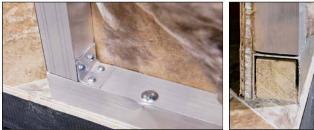
All aluminum sills and wall studs are mechanically joined and the aluminum sill tubing is fully reinforced internally with wood, providing greater strength and stability when it is "bolted-through", never screwed, to the sub-floor structure and the steel frame below.
