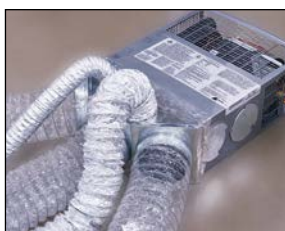
High density wool insulation blankets the underbelly frame spaces and the flooring assembly, to provide added protection for the water systems. Perimeter heating features 6" ducts and custom plenum with 5-duct heating.
