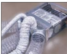
High density wool insulation blankets the underbelly frame spaces and the flooring assembly, to provide added protection for the water systems. Perimeter heating features 6" ducts and custom plenum with 5-duct heating.
