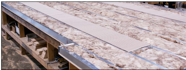
High density wool insulation blankets the underbelly frame spaces and the flooring assembly, to provide added protection for the water systems. Perimeter heating features 6" ducts and custom plenum with 5-duct heating.
